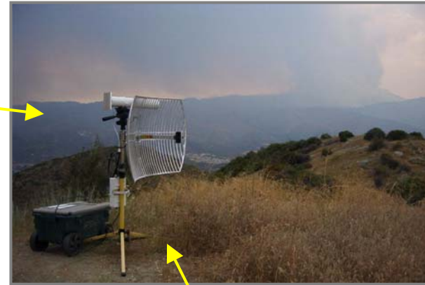
Line-of-sight radio relay site
