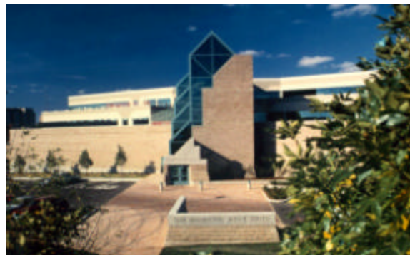
Figure 20. AHPCRC systems are located in this state-of-the-art building specifically designed to protect and support HPC systems and operations.
