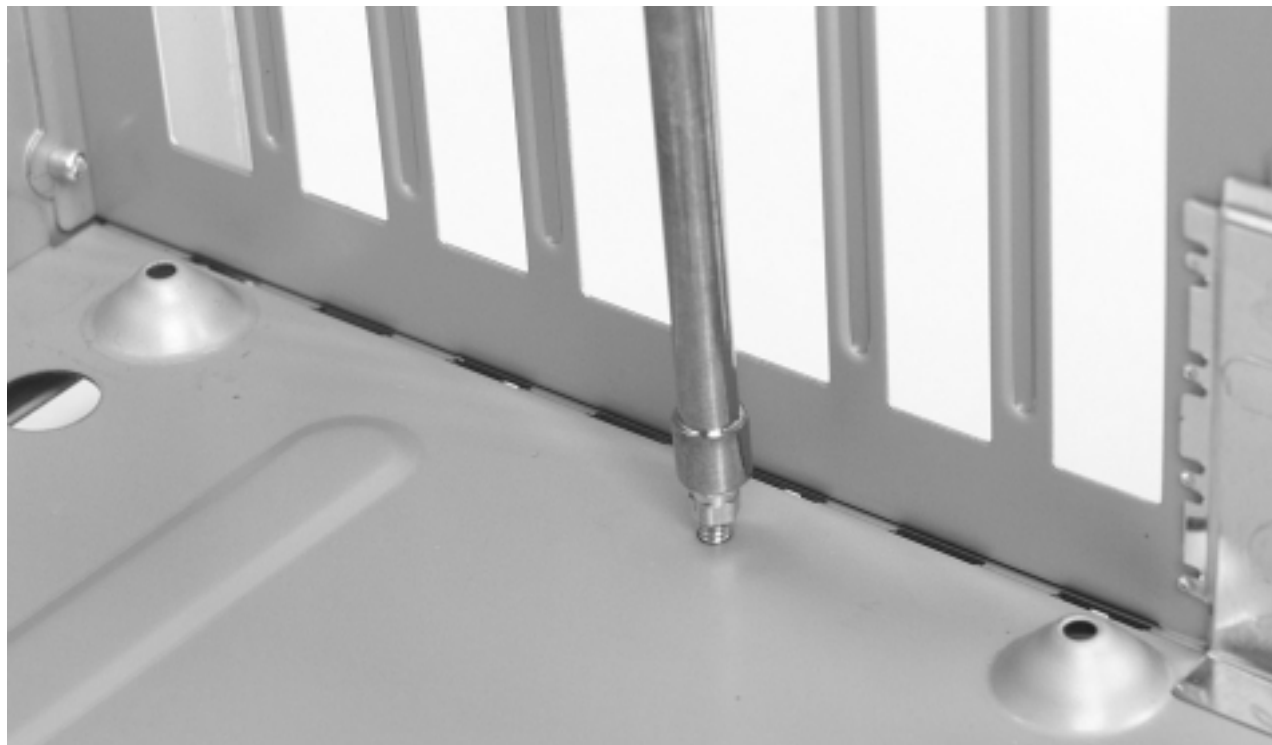
Photo 25. Installing the Extra Standoff
